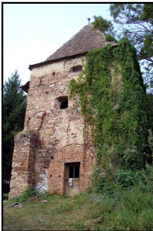
Fig. 2.07.4: East gate tower with bricked portcullis.
