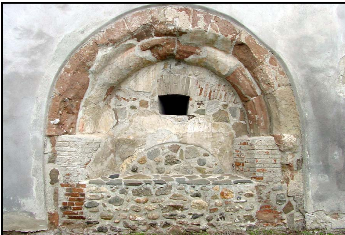
Fig. 2.43.5: South side view of the bell tower wall with Romanesque arch bricked up in 1495.
