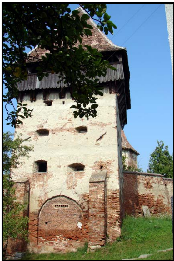
Fig. 2.06.3: Gate tower with bricked up portcullis and battlements.
