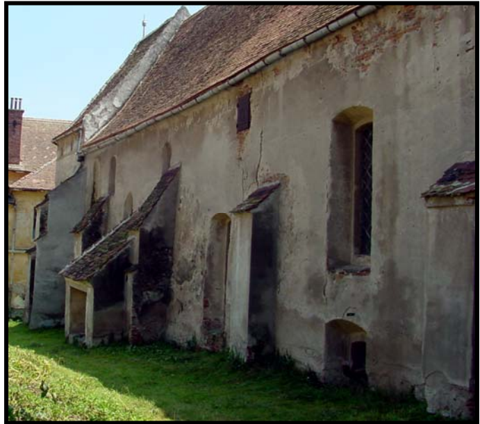
Fig. 2.125.2: View from the northwest of Șeica Mare church with north entrance portal and external prop columns.
