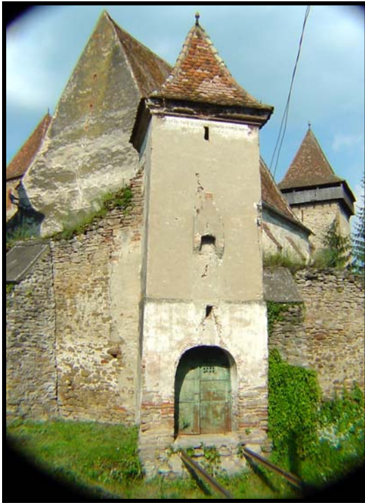
Fig. 2.152.3: Southeast view of the personnel gate tower with casting oriel and remnant of the moat surrounding the complex.
