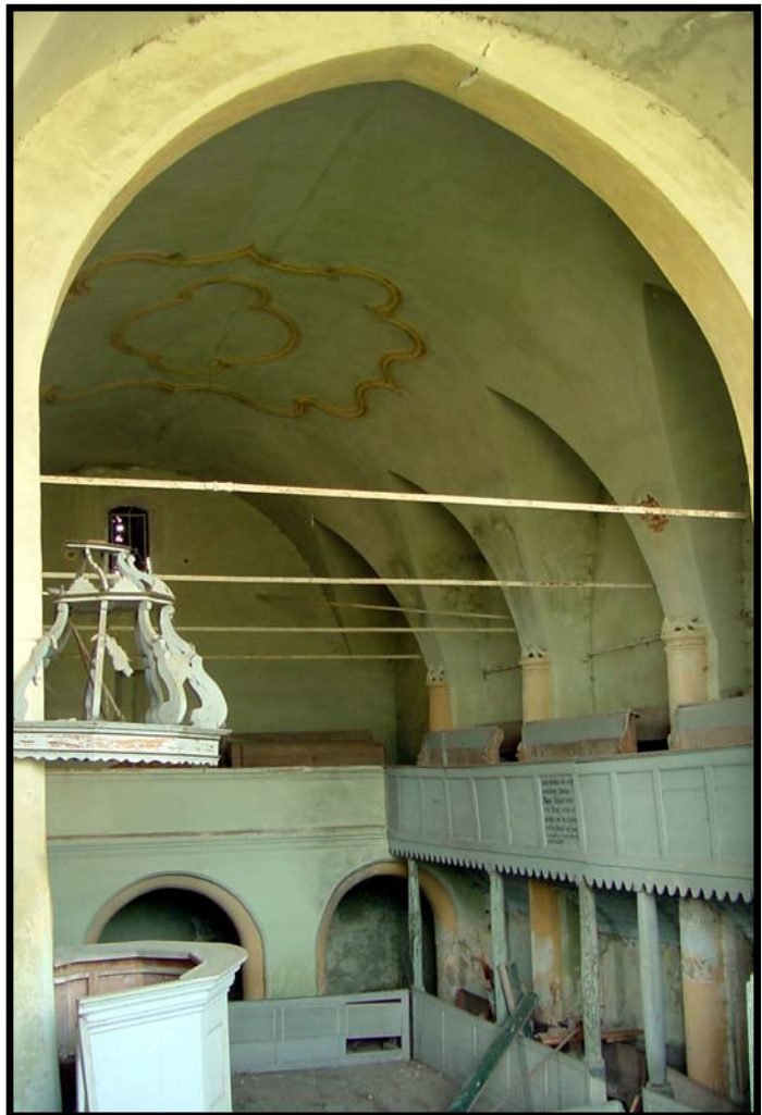
Figure 6.23: Velt – ruined nave from the east showing the patron's gallery and blocked up windows above along the west tower wall.
