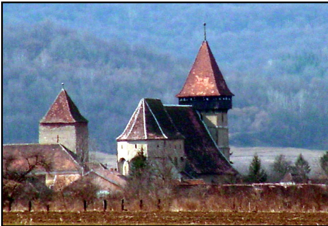
Fig. 2.26.3: View from the south of the Bratei church and the south-west tower. Note the external prop-columns supporting the military fortified choir.
