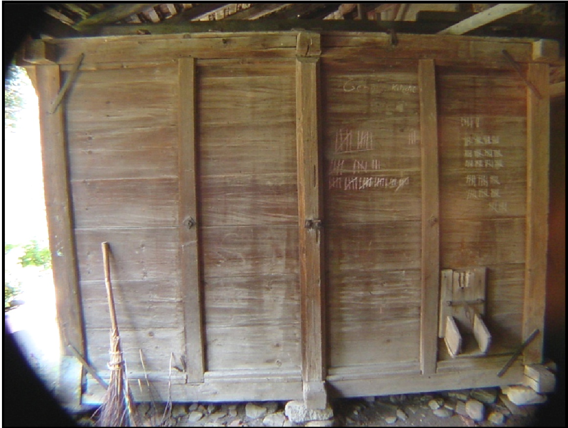
Figure 5.44: Miercurea Sibiului: movable communal storage bin for wheat with dispensing chute, rebuilt several times. Documents indicate the bin dates from the mid-fifteenth century.
