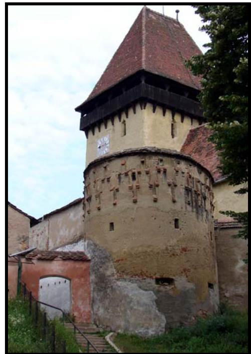
Fig. 2.67.4: (Above right) detailed view from the southeast of the circular bastion with visible shooting loopholes.
