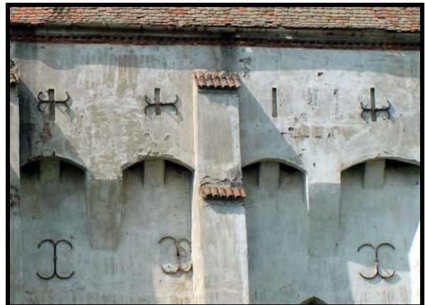
Fig. 2.22.1: View of Boian's choir showing casting oriels and prop columns.
