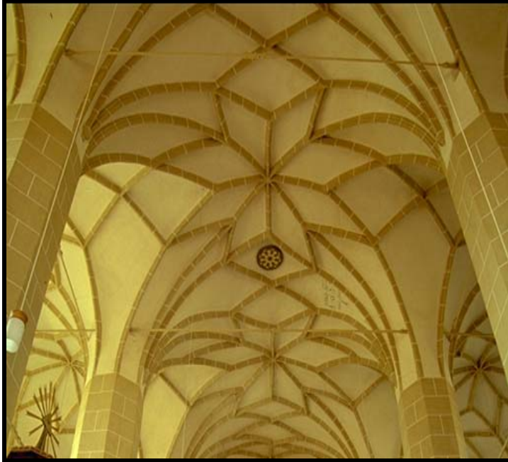
Figure 6.13: Sex-partite vault of Biertan nave.
