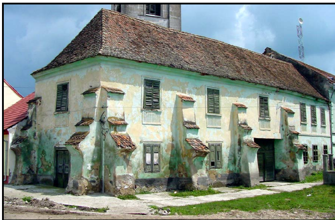
Fig. 1.45.3: View of the Mercheaşa church chapter house built into the outer precinct wall and its external prop column buttresses.
