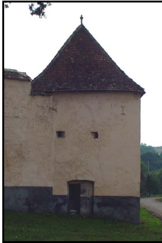
Fig. 2.27.2: The north precinct wall and corner bastion with loopholes.
