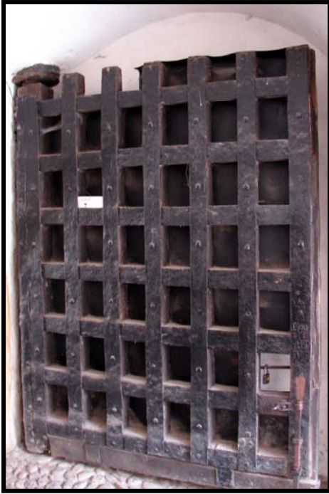
Figure 7.19: Prejmer portcullis dating from 1501 with original iron strapping.
