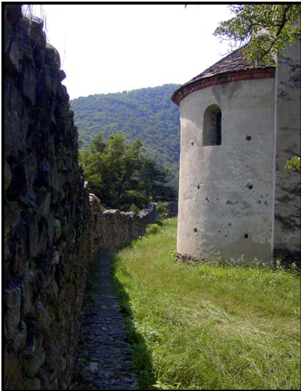
Fig. 2.37.5: View from the north of the remains of the flush gate tower along the south wall and the crenellations and merlons built into the precinct wall.
