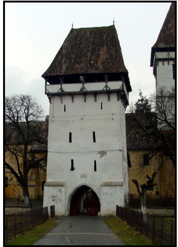
Fig. 2.03.4: (Above right) cooper's or Faßbinder tower, arrow loops and portcullis.
