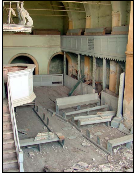
Fig. 2.157.4: Detailed view of the collapsed choir with interior wood furnishings dating from the 1500s. Note the unusual square columns that support the roof and walls.
