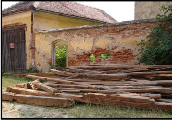
Fig. 2.90.3: (Above) view of the northwest tower oak beam renovation with timber removal dating from the mid 1500s.
