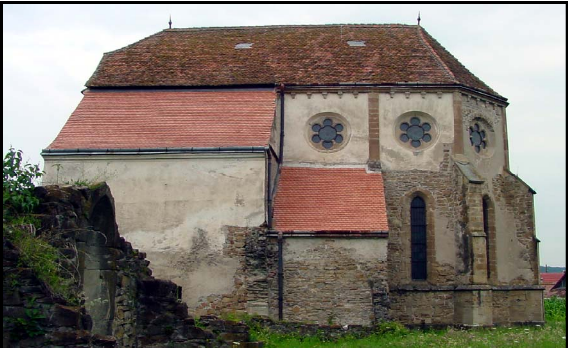
Fig. 2.35.3: View from the south of the present Cîrța church showing the six rosette windows around the polygon shaped choir of the original transept and choir.
