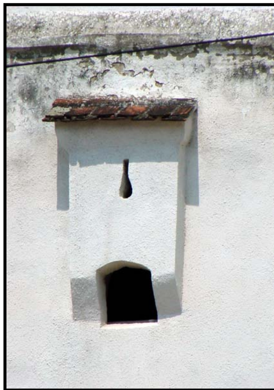
Fig. 2.80.3: Detailed view of a shooting loophole and casting oriel.
