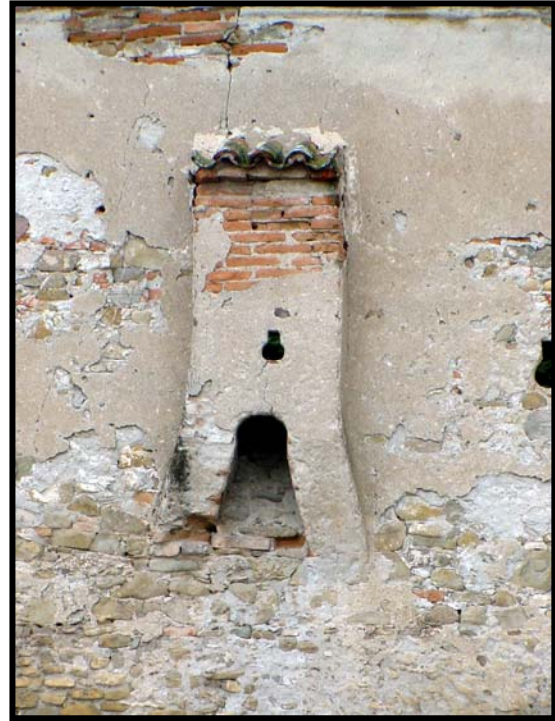
Fig. 1.53.4: View of Rotbav (Rothbach) precinct wall defensive works including a casting oriel or Gußerker.
