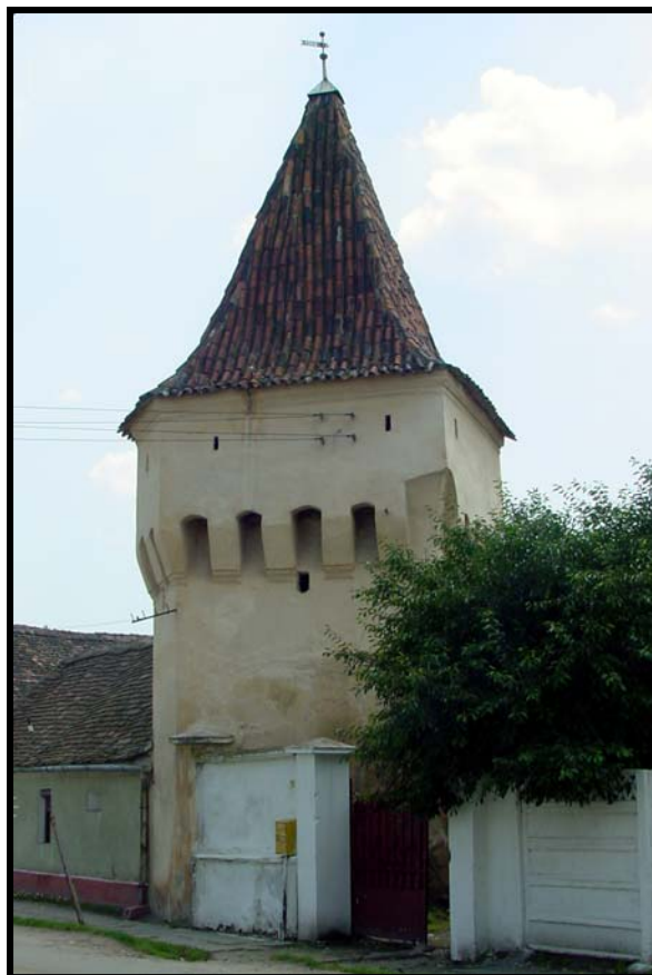
Fig. 2.146.3: (Right) view from the east of the hexagon tower with details of casting oriels.
