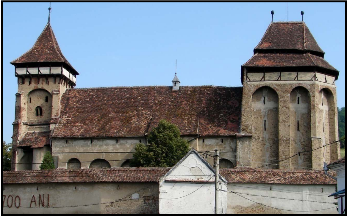
Figure 5.26: View of Valea Viilor fortified church with the stone machicolated platforms on external prop columns extending over the choir, west tower and the side aisles of the church.
