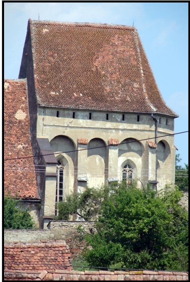
Figure 5.17: Copşa Mare church with external prop columns or buttresses used to reinforce the walls with machicolations between the columns of the choir.
