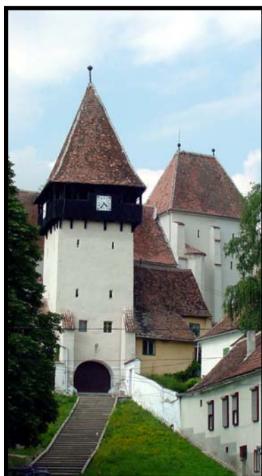
Fig. 2.16.3: South gate and bell tower with portcullis and combination bretèche and machicoulis.
