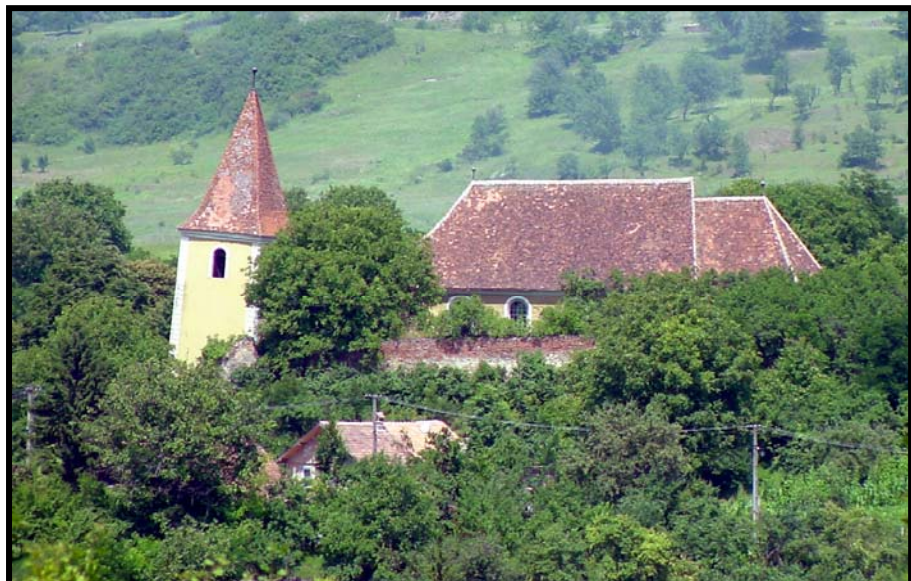
Fig. 2.116.1: View from the southeast of the church complex with tower clearly out of vertical.
