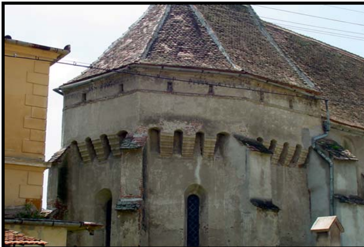
Fig. 2.125.3: View from the northeast of the defensive elements of the choir with the defensive floor elements.
