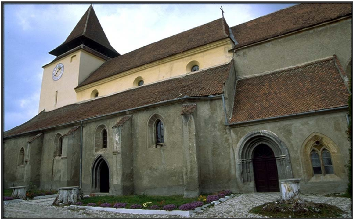
Fig. 1.32.3: Ghimbav church showing the stages of building with the original Romanesque form and Gothic alterations.
