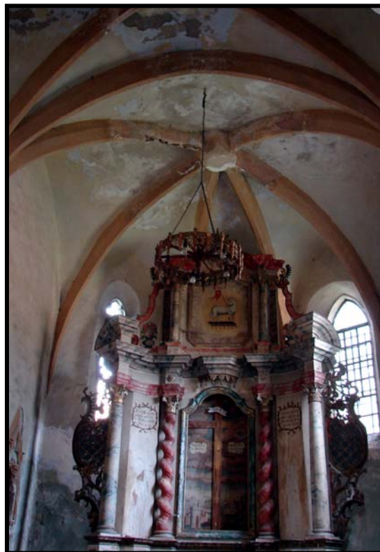
Fig. 2.30.5: Interior view of the church choir damage due to water seepage.
