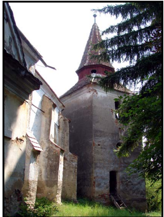
Fig. 2.162.3: View from the southwest of the donjon bell tower with octagonal defensive roof on a wooden pyramid base.
