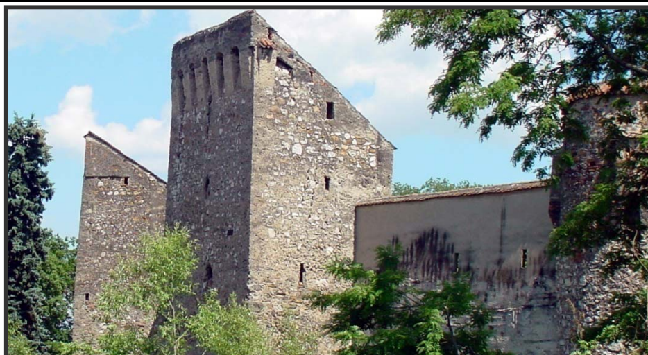
Fig. 1.19.1: View of the exterior of the precinct wall with mono pitch defensive towers and oriel.
