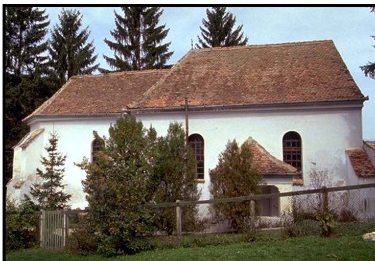
Fig. 2.111.2: View from the north of the hall-style church with external prop columns and the 5/8 th size choir.
