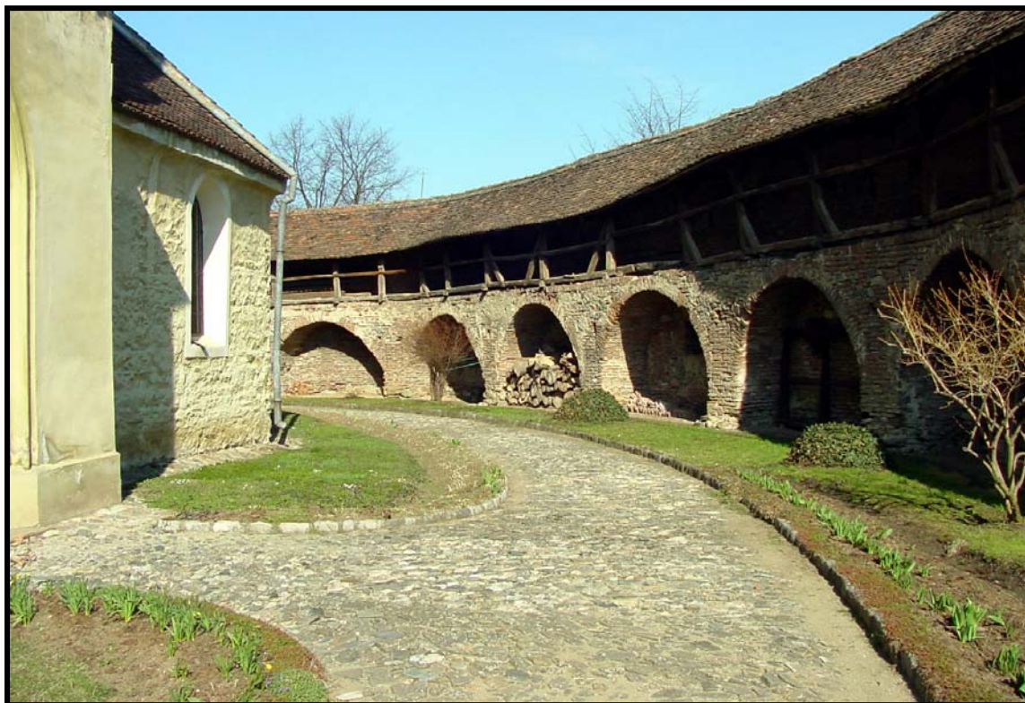
Fig. 2.36.6: Interior view from the west of the church precinct wall showing the covered allure built over arched brick arcades storage compartments for villagers.
