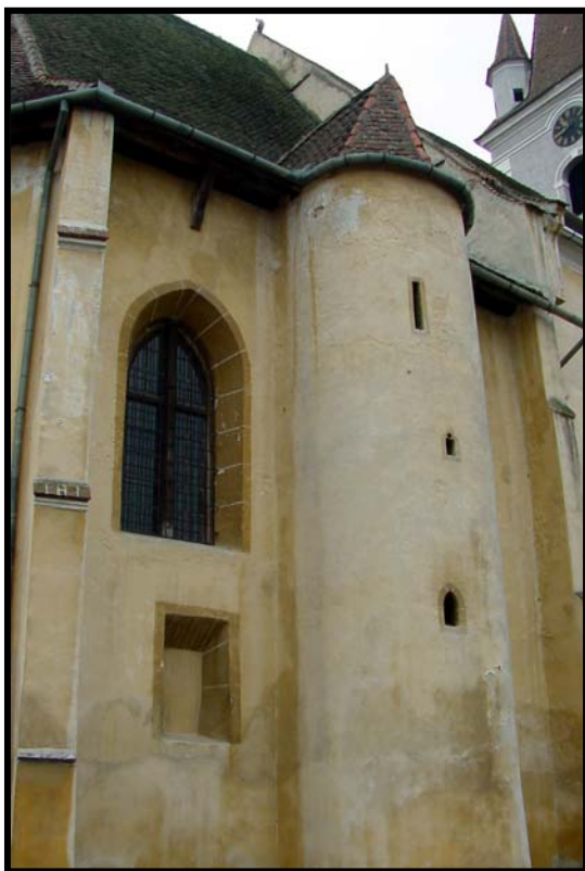
Fig. 2.43.3: Northeast view of the choir and staircase with loopholes.
