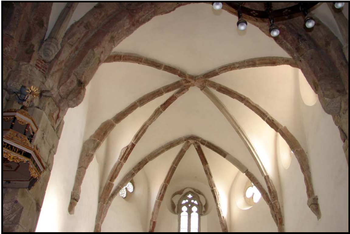
Figure 7.30: Prejmer church north transept with Cistercian Gothic ribbed vaulting on corbelled piers.
