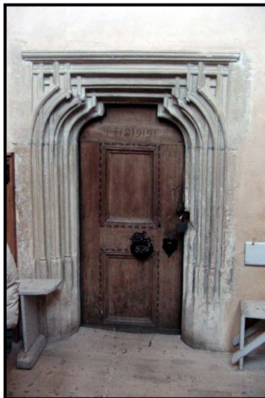
Fig. 2.13.6: Gothic doorway and fasteners.
