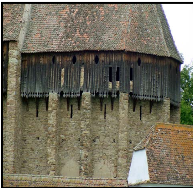
Fig. 2.24.4: View from the southeast of the Brădeni fortified choir with intact battlements built into the raised choir of the church.
