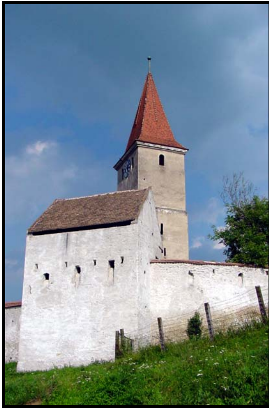
Fig. 2.122.3: View from the northwest of the precinct wall and northwest tower with plunging and arrow loopholes.
