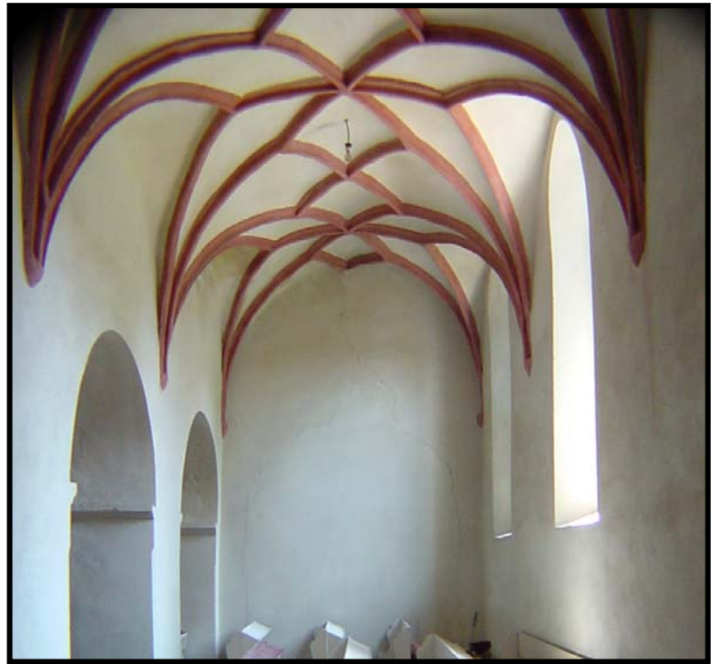
Figure 6.12: Quadri-partite vault in east aisle of Ocna Sibiului.
