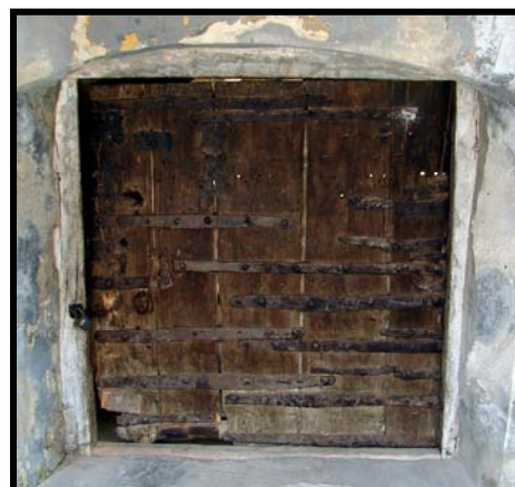
Fig. 2.86.1: View from the south of the fortified door entrance along the south precinct wall below the school with medieval iron strapping.
