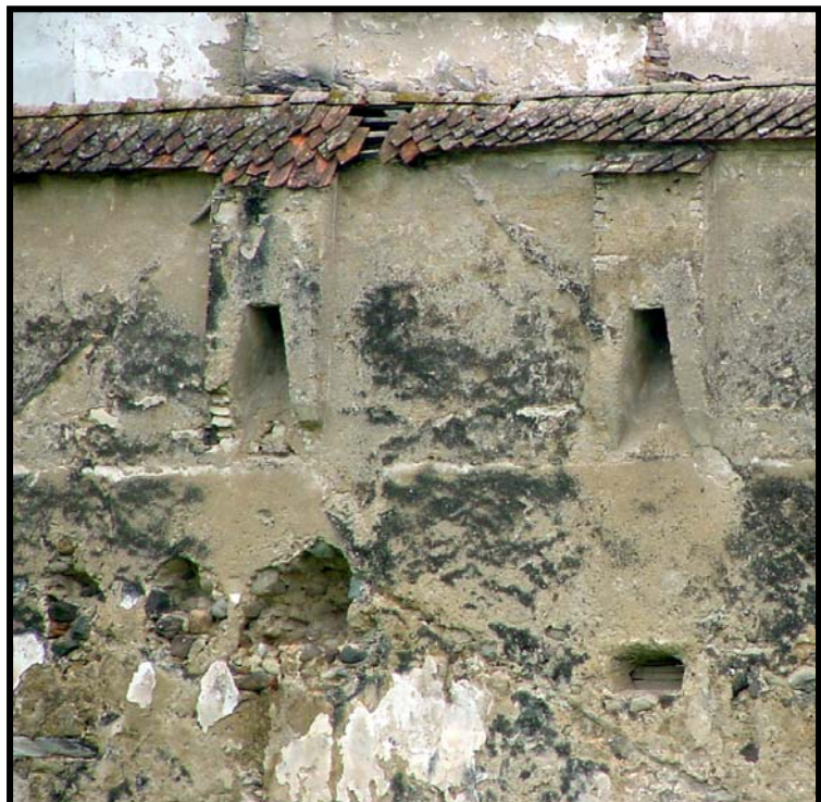
Fig. 1.45.1: Close up view of the Mercheaşa outer precinct wall showing the casting oriels.
