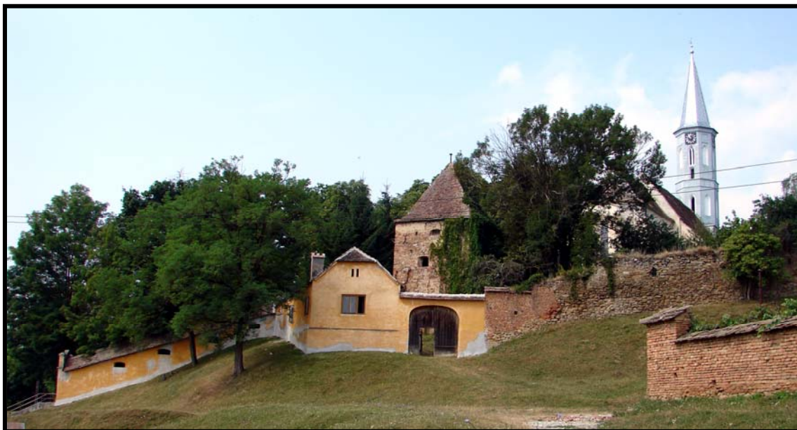
Fig. 2.07.2: Gate tower with bricked up portcullis and battlements.
