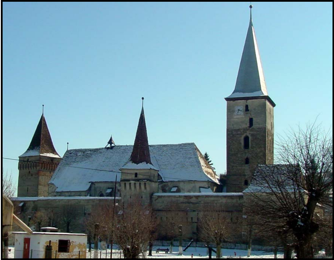
Figure 5.28: Moșna curtain wall with corner and recessed mural towers, note the hall church and separate west donjon / bell tower.
