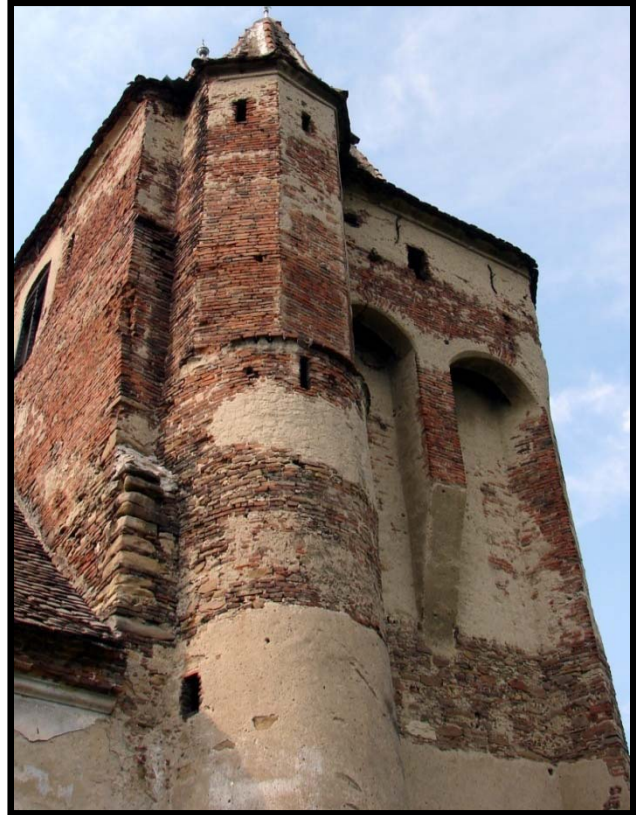
Figure 5.19: Buzd donjon church tower with external circular stairway and machicolations.
