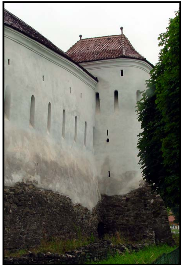
Figure 7.23: Original walls of Prejmer made of river stone with tuff addition shown in white.
