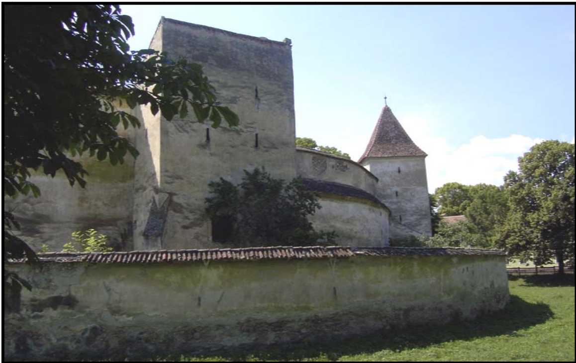
Fig. 1.36.4: Exterior view of the double precinct wall at Härman and different types of towers and moat depression.
