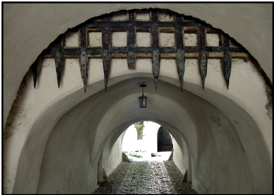
Figure 5.43: Prejmer -- third portcullis with machicolation behind followed by last door.
