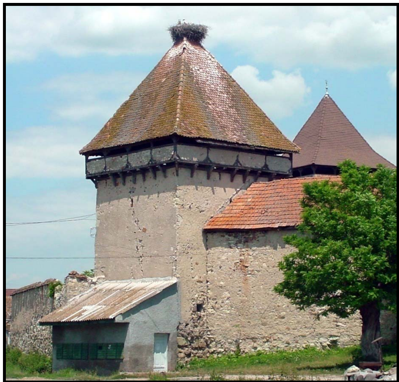
Figure 5.31: Caţa outer precinct wall with recessed mural tower complete with battlements and wall walk.
