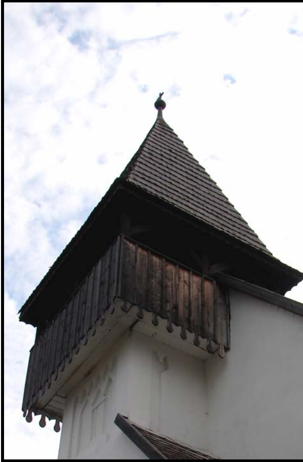
Fig. 2.40.2: Detail of the west-front Romanesque bell tower fortified with a battlement and defensive pyramidal roof.
