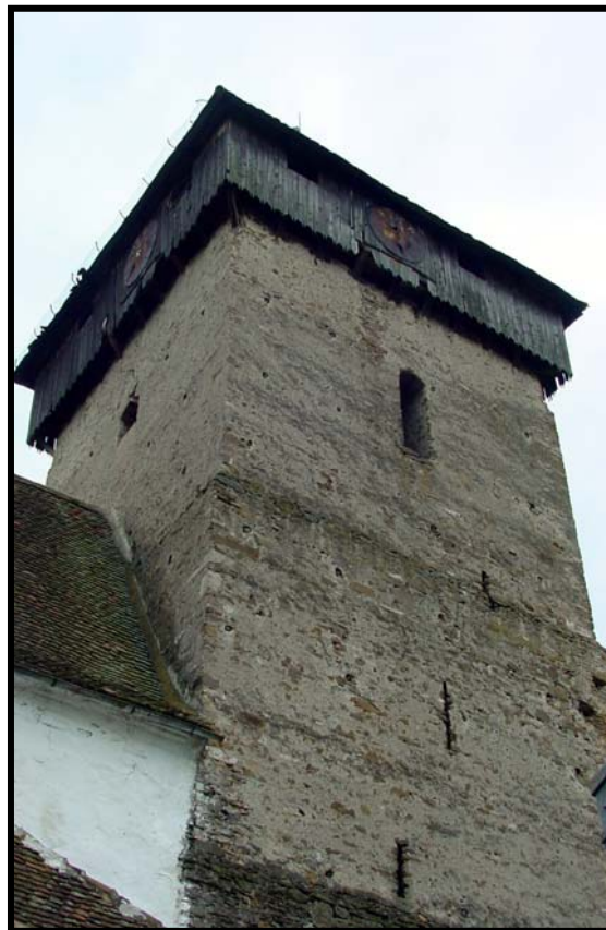
Fig. 2.114.3: View from the south of the church donjon tower and battlements made of stacked river stones.
