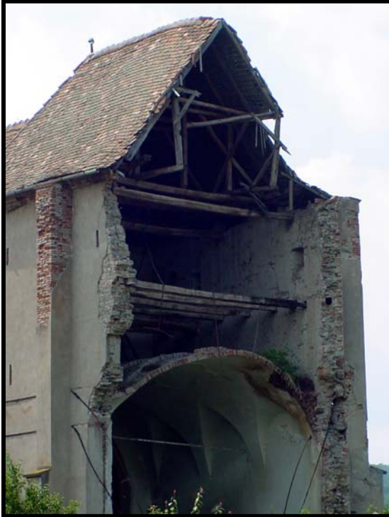
Fig. 2.157.3: View of the collapsed choir from the southeast with exposed defensive floors installed above the vaulting.
