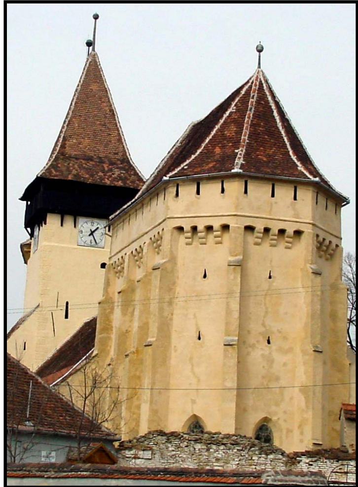
Figure 5.27: The fortified choir at Seica Mică with loopholes and corbelled machicolated hoardings.
