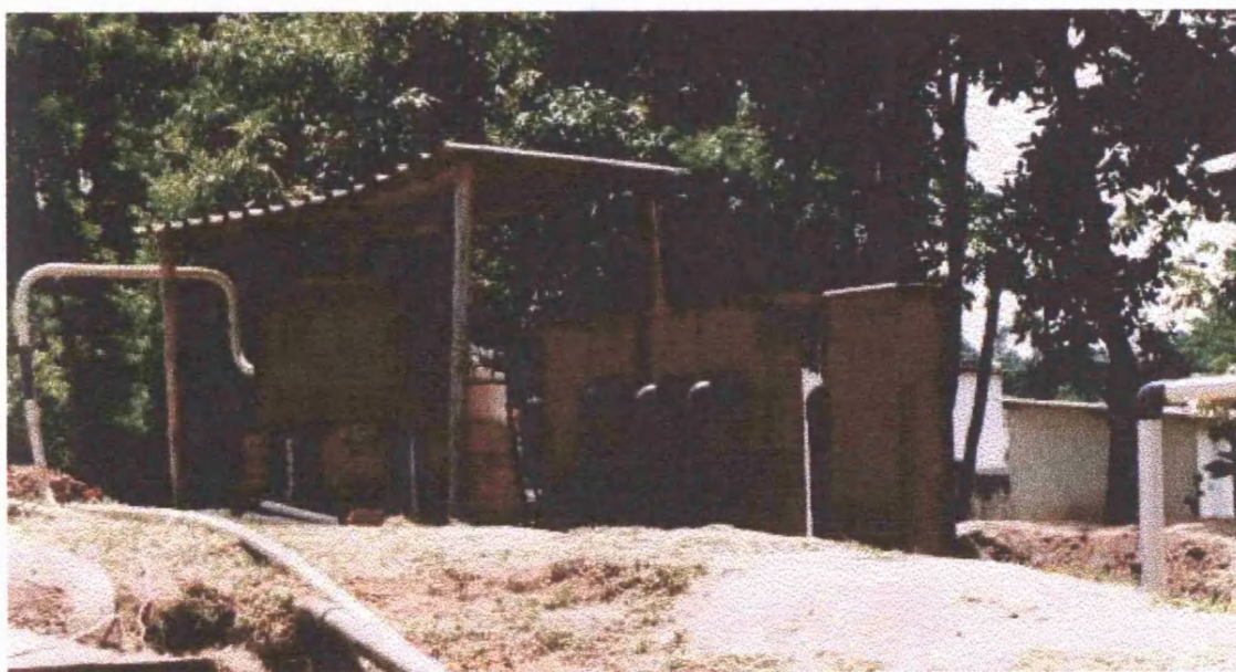
Figure 5.17 Photograph showing header tank and modified flocculation units
