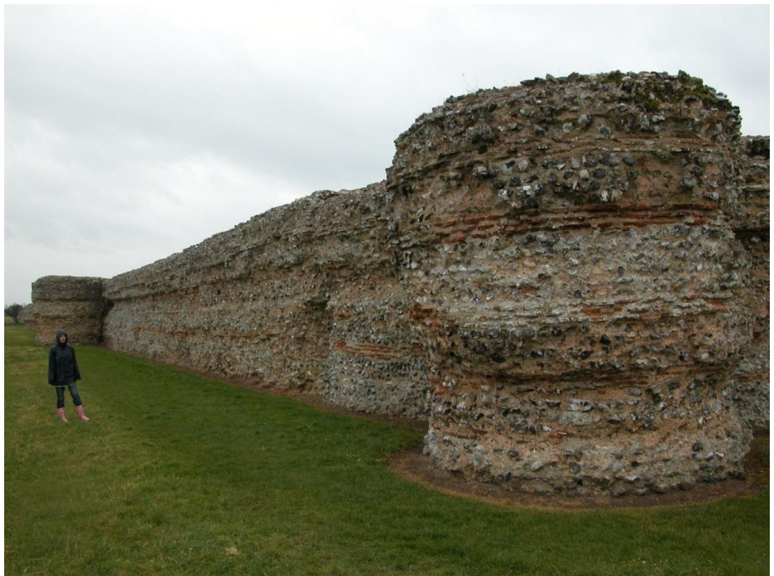
Figure 101: External projecting towers at the Saxon Shore Fort of Burgh Castle, Norfolk, built AD 280-300 (photo by author)
