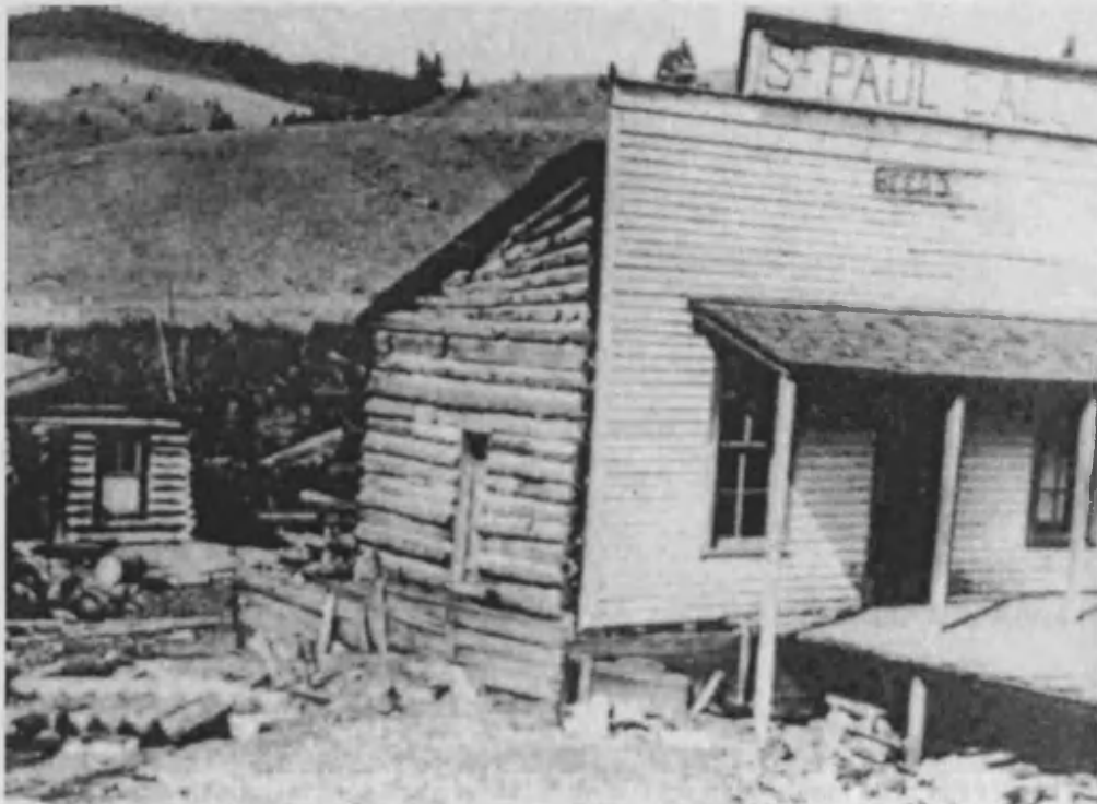
Fig. 1.2: A log saloon in Unionville, MT, 1870s. Note the simple long construction with a planking veneer added to give the impression of a timber framed building (from West 1979, 38)
