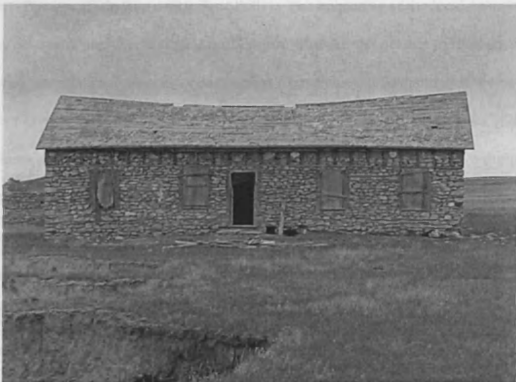
Fig. 1.4: Ackerman Homestead, Garfield County, Montana. This homestead, built c. 1910, in some ways was an exception. Located in an area where timber was extremely scarce and the sandy soil made the production of sod brick difficult, the pioneers used readily available sandstone outcroppings to construct their buildings. Thus, while the final product was a stone building, the behavior pattern was consistent with the use of locally abundant natural resources with minimal financial investment (author's personal collection).
