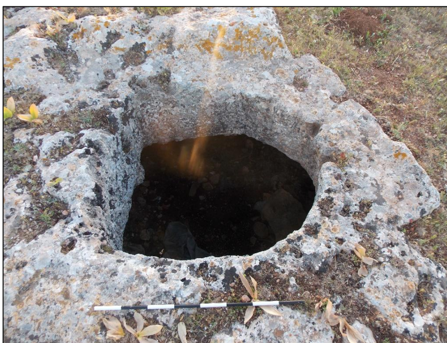
G 102: The horseshoe-shaped opening of the water cistern, looking east (Author).
