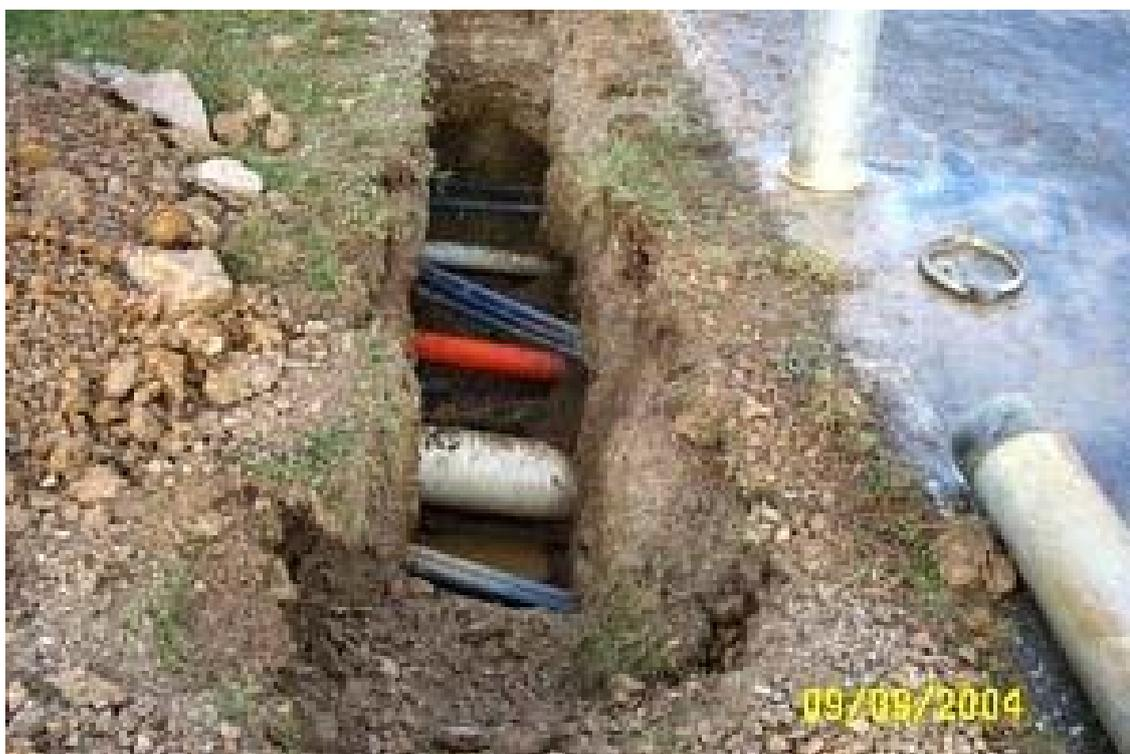
Figure 3.2: Excavation of underground cables
