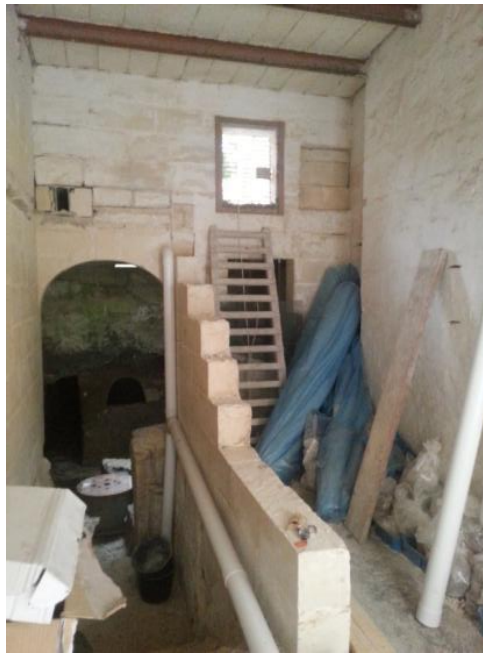
Figure 4.5 – The entrance to Saint Augustine’s Catacombs extended by demolishing a dividing wall (source: Author)
