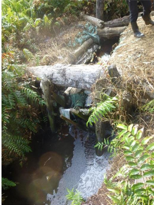
**Figure 2.9.** Example of wooden weir structures located in the SE main drain, used to artificially modify water channel heights.
