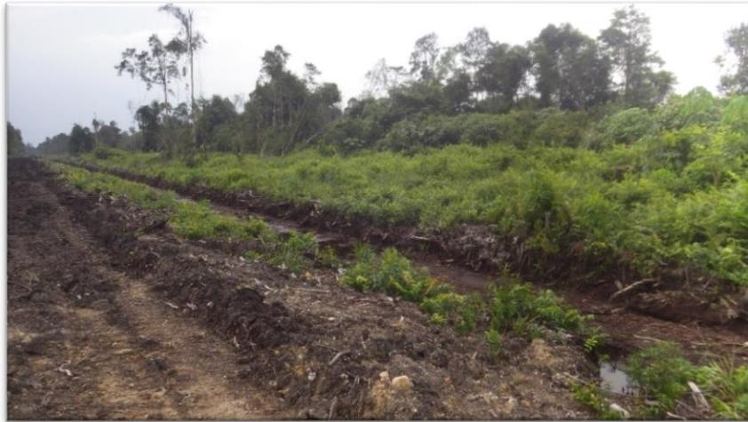
**Figure 2.22.** The 3 m drainage ditch within the DF site, approximately 3 m wide and 2 m deep
