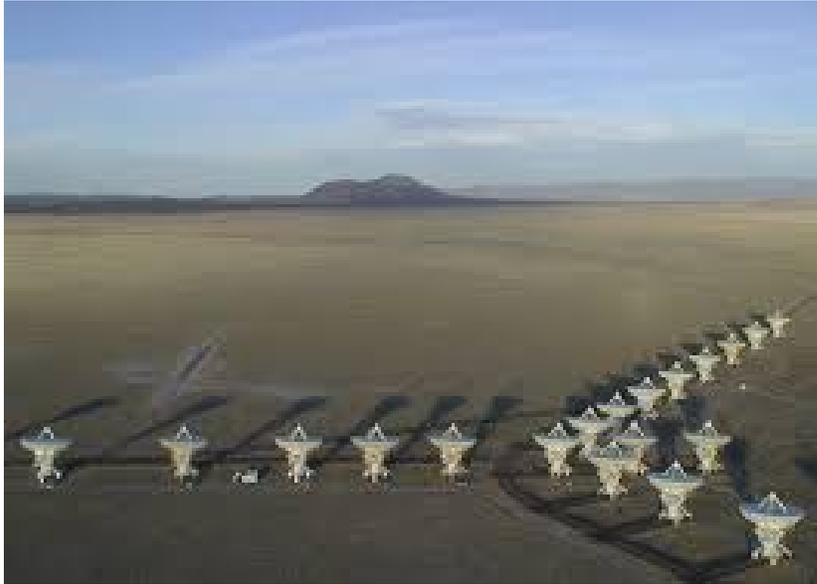
Figure 2.7: Image, taken from Perley et al. (2011), illustrates layout of the array of antennae, showing the Y-distribution used to produce the baselines.
