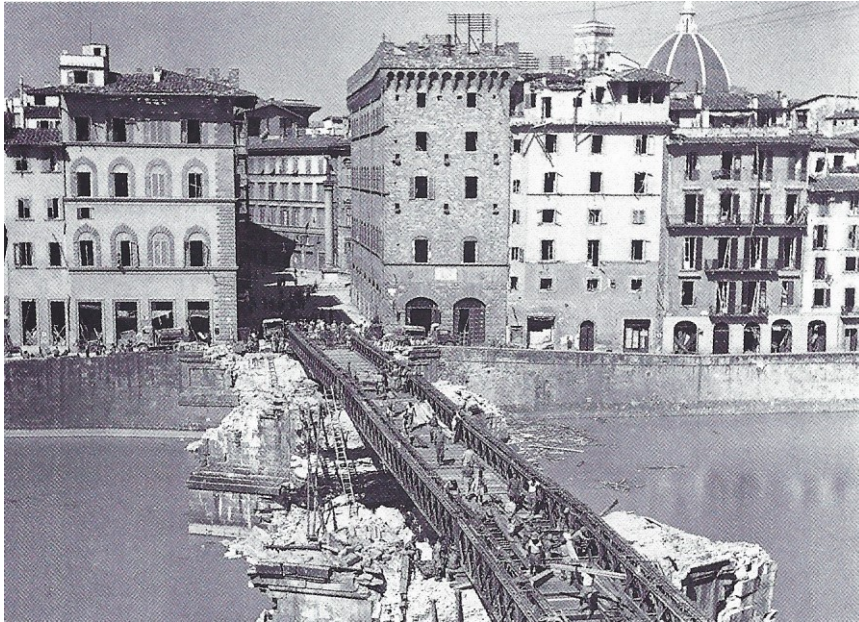
Figure 40 - Picture of the Bailey bridge built by the Allies on the ruins of Ponte Santa Trinita (Florence), destroyed by the Germans on the night between the 3 rd and 4 th of August 1944.
